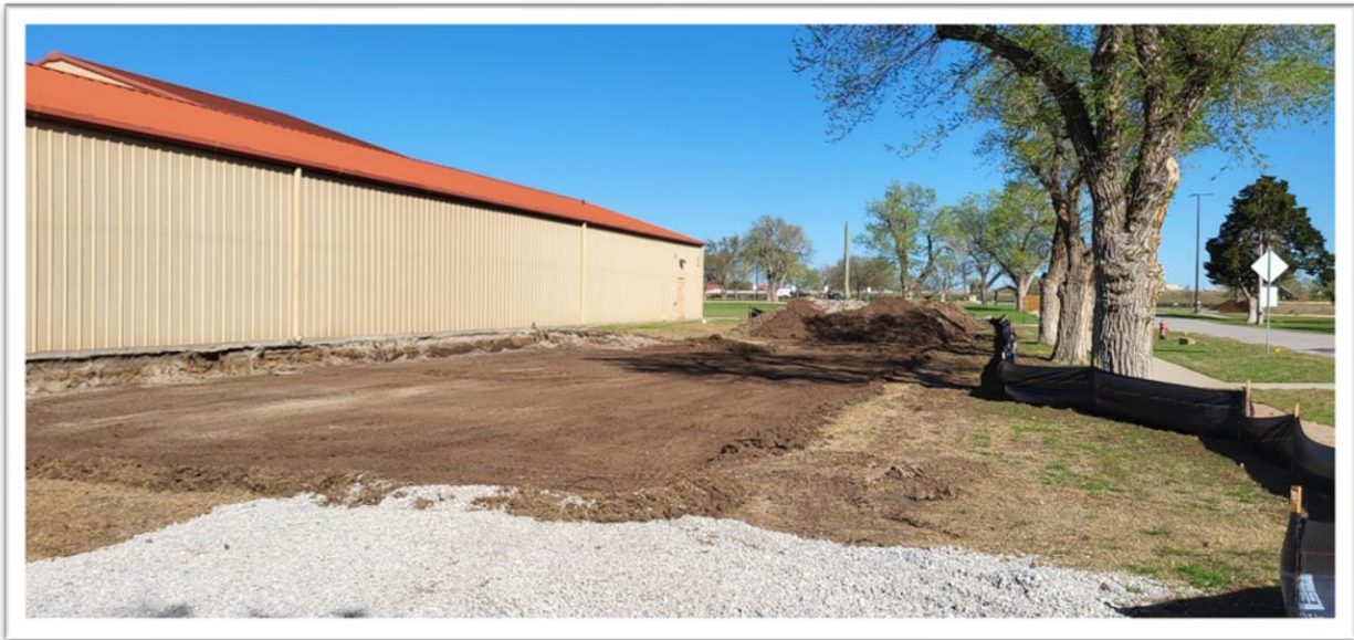
Future home of the Artillery OCS Heritage Hall 40'x 80' addition and 40' x 50' courtyard attached to the South Gallery of the US Field Artillery Museum at Fort Sill. (March 2023)
