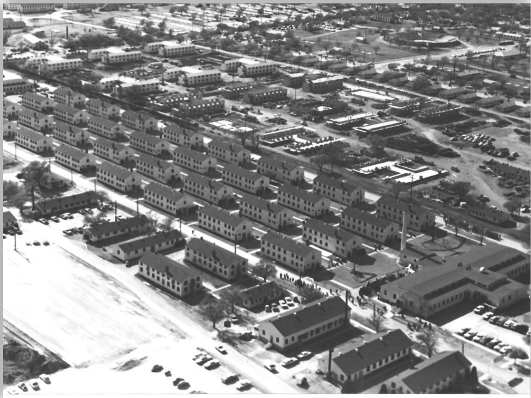
Robinson Barracks during 1966-1967 Expansion
