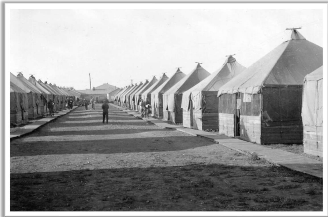
The first Field Artillery OCS candidates were billeted in 6-man pyramidal tents. In 1942 the area was converted to 6-man tarpaper and frame Hutments.
